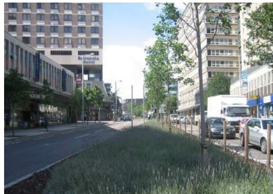
Incorporating street trees and planting into the streetscape (Maid Marian Way, Nottingham)
