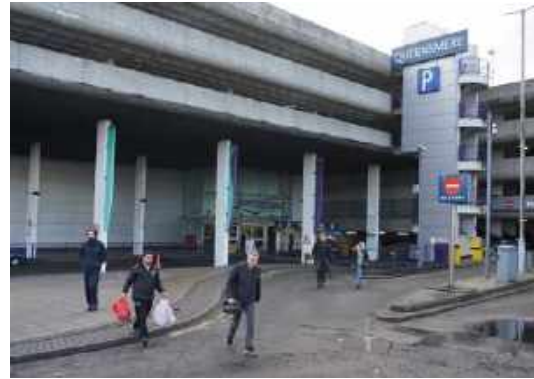
Inhospitable walking environment at the entrance to the Queensmere Centre on Wellington Street
